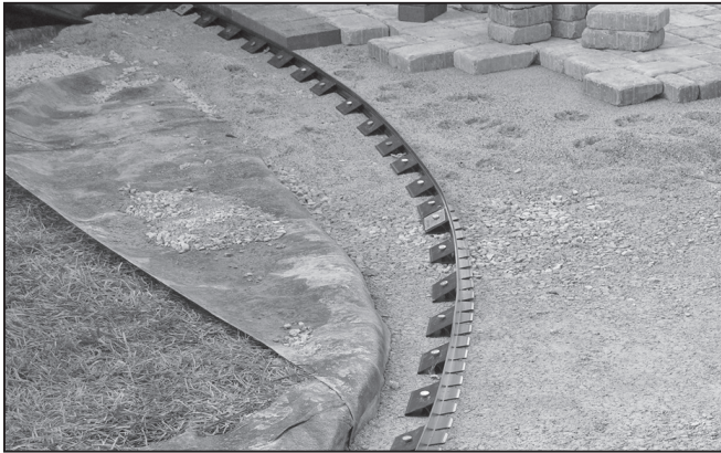
Install edge restraints.
