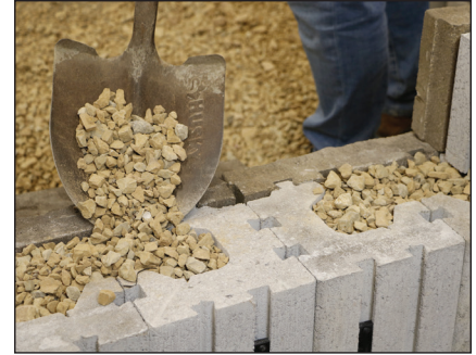
Diagram 5—Fill cores with free draining aggregate
