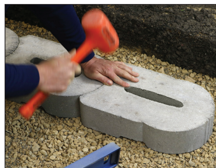
Diagram 19—Lay and level base block
