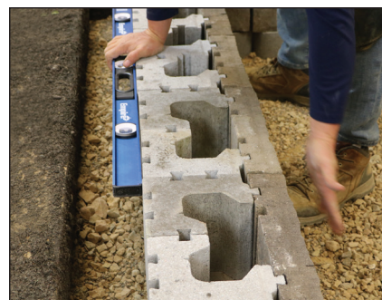
Diagram 4— Assembled units on top of U Start block
