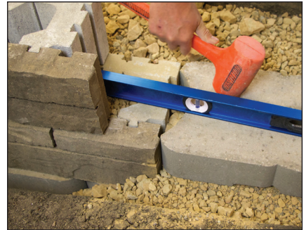
Diagram 7—Stepping up the base
