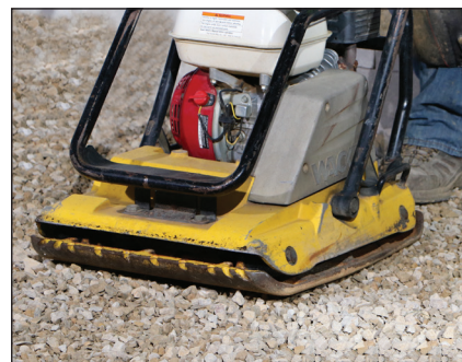
Diagram 2—Leveling Pad
