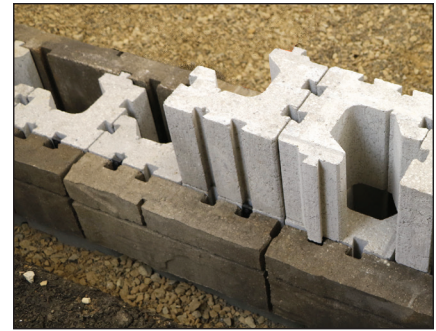
Diagram 21—Second course construction
