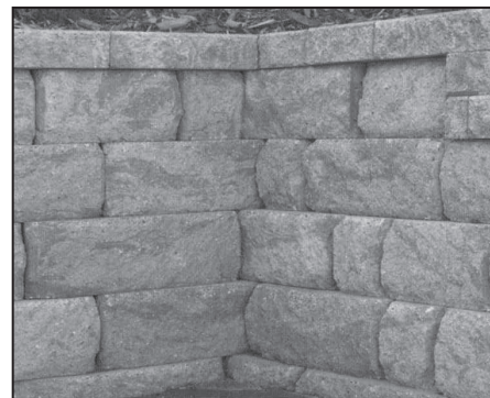
Example Inside 90-Degree Corner
