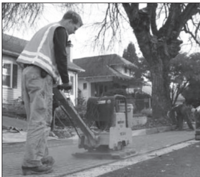
PICP paver compaction shows that pavers need to be set about 3/4-inch (19 mm) above their final elevation before compaction and 3/8-inch (10 mm) after compaction to account for downward movement.
