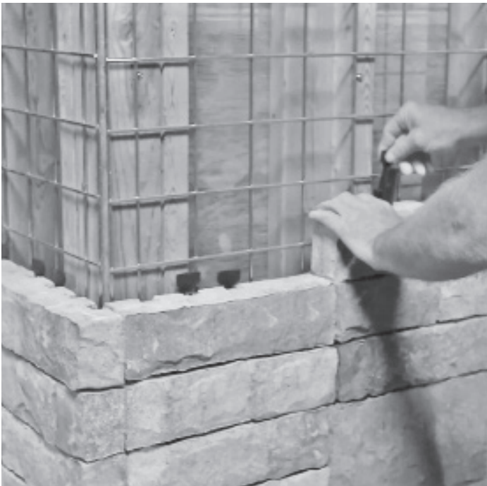
Attach Lafitt Tandem Veneer with Connector
