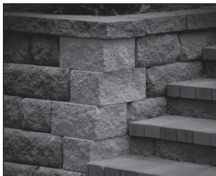
Outside 90-Degree Corner with Corner/Column Unit
