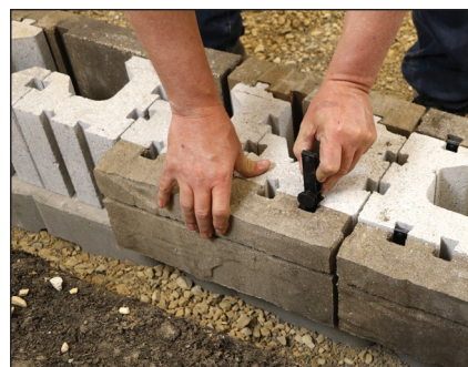
Diagram 20—Placing veneers onto modular block
