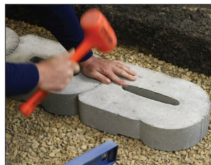
Diagram 3—Lay and level base block
