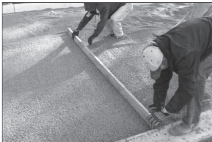
Manually screeding the No. 8 stone setting bed.
